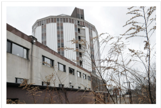
Former Monsour Hospital Photo credit: Bob Donaldson/Post-Gazette
